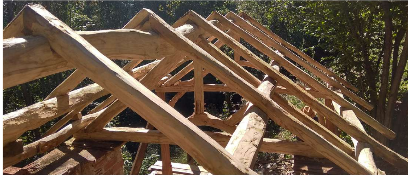
Photo 1 | On-site timber frame installation
