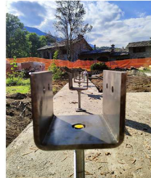
Photo 4 | Steel base plate detail
