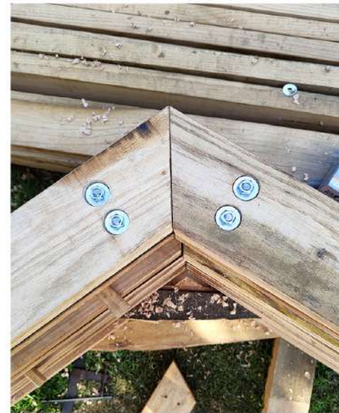
Photo 3 | Ridge joint detail
